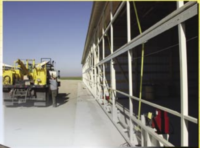
Schweiss Installation Progress
